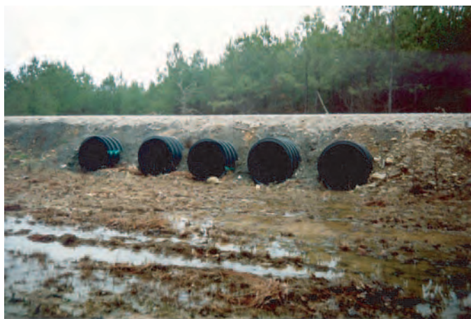
Figure 5-1. Example of multibarrel culvert installation.
