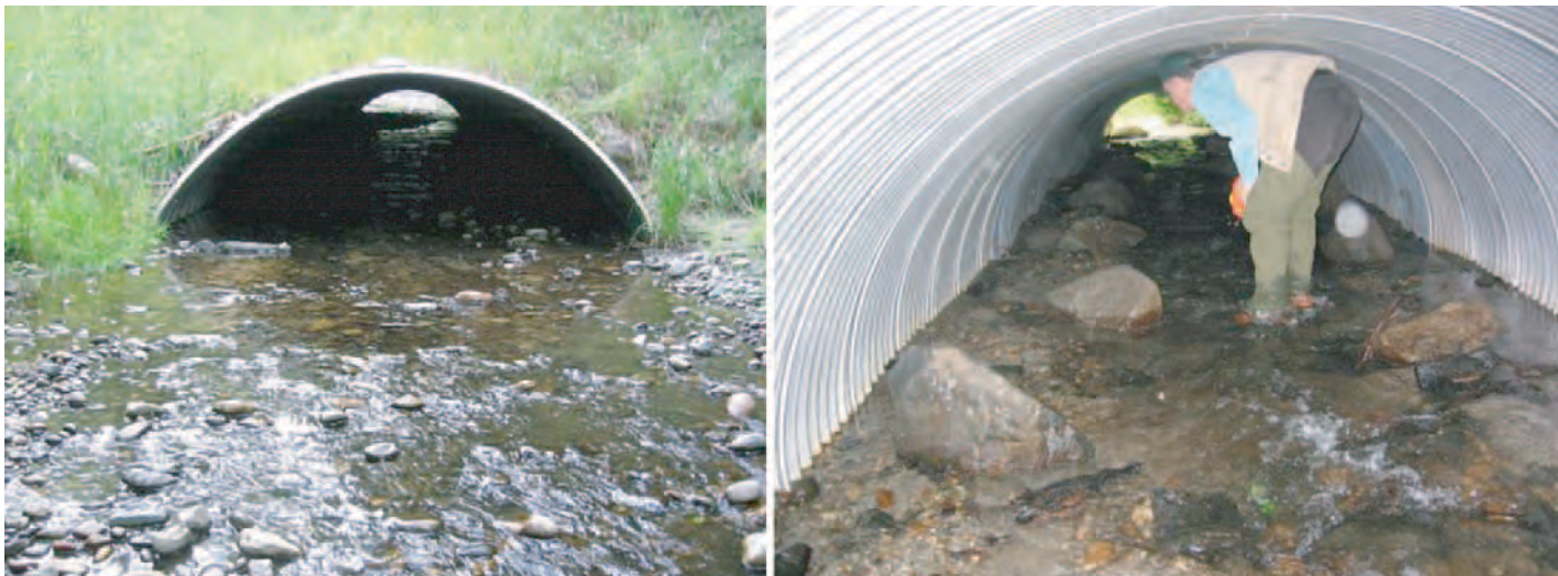
Figure 2-1. Examples of buried-invert culverts for fish passage.
