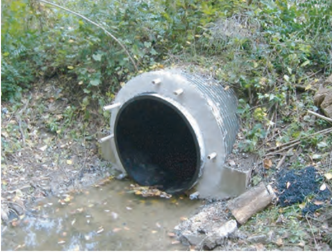
Figure 3-1. Example of a slip-lined culvert.
