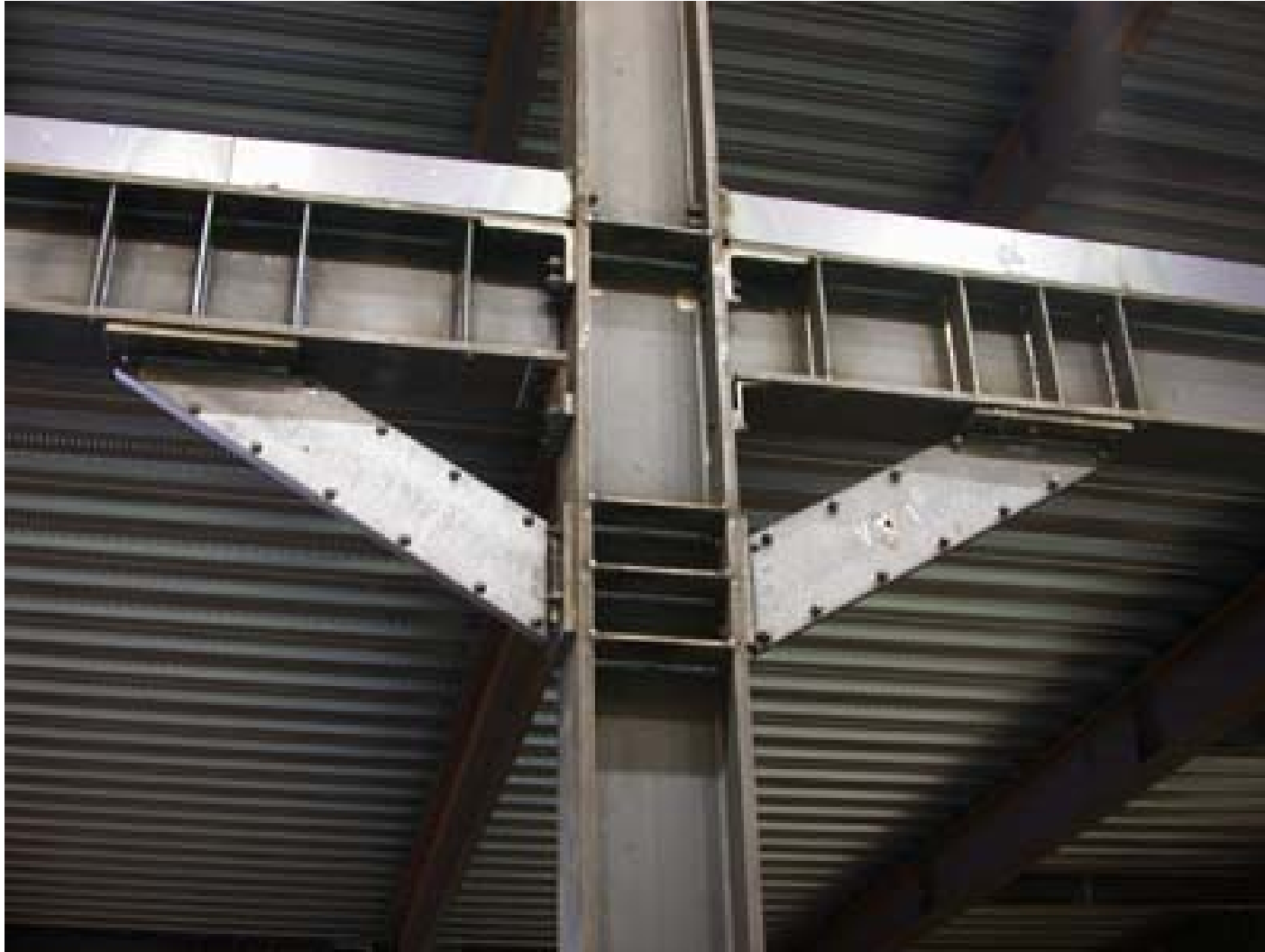
Earthquake Resistant Connection
