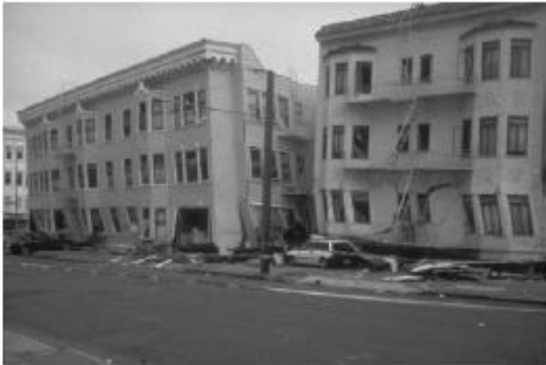
SOFT STORY FAILURE
