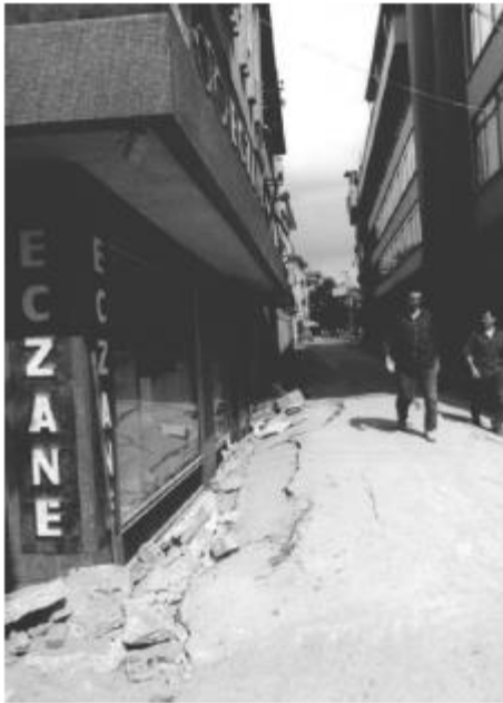
BEARING CAPACITY FAILURE
