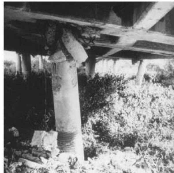
PILE FAILURE
