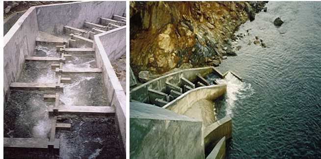
Fig. 3.5 – Fish-ladders of pool-type with bottom orifice and top weir.
