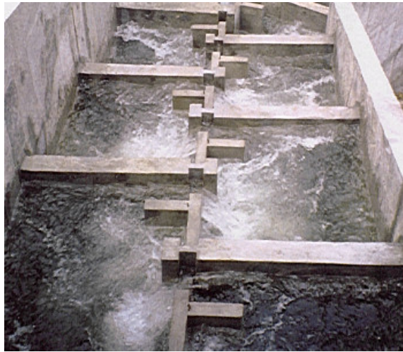
Fig. 9.2 – A fish-ladder of a SHP.
