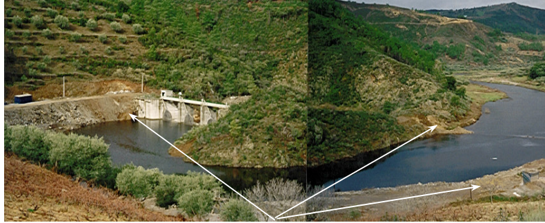
Fig. 3.4 – Visualisation of the dry zone to absorb floods.
