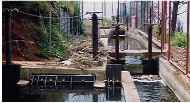
Fig. 3.2 – Diversion canal for a powerplant.
