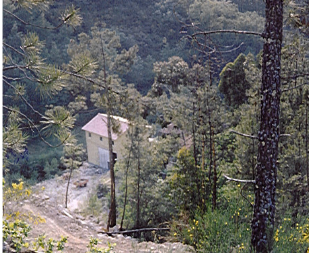
Fig. 9.4 – An example of a SHP powerhouse in landscape integration.
