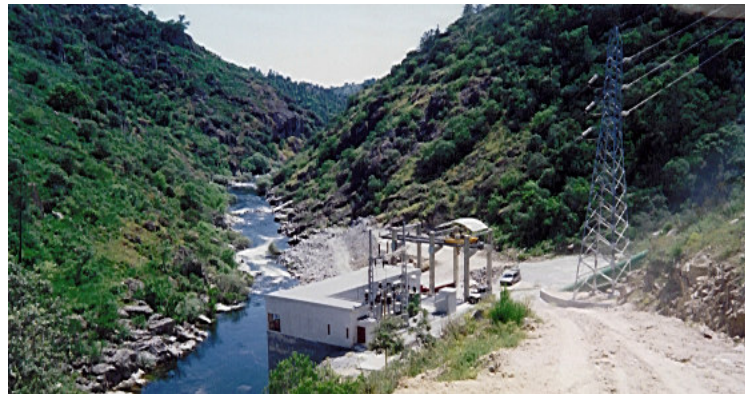
Fig. 8.9 – Grid substation to transform the energy produced from 6kV to 60kV and fed it into the supply network of the national electric grid.
