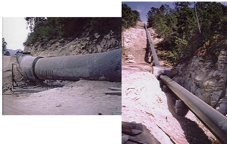
Fig. 9.5 – Deforestation for pipe installation.
