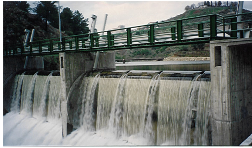
Fig. 2.1 – Typical scheme of dam used to raise head for intake diversion and small water storage.
