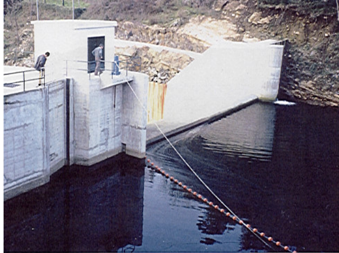
Fig. 9.7 – A life guard grid with float balls.
