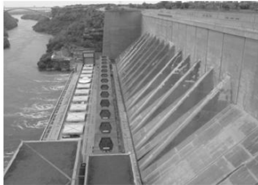
Niagara Hydroelectric Dam
