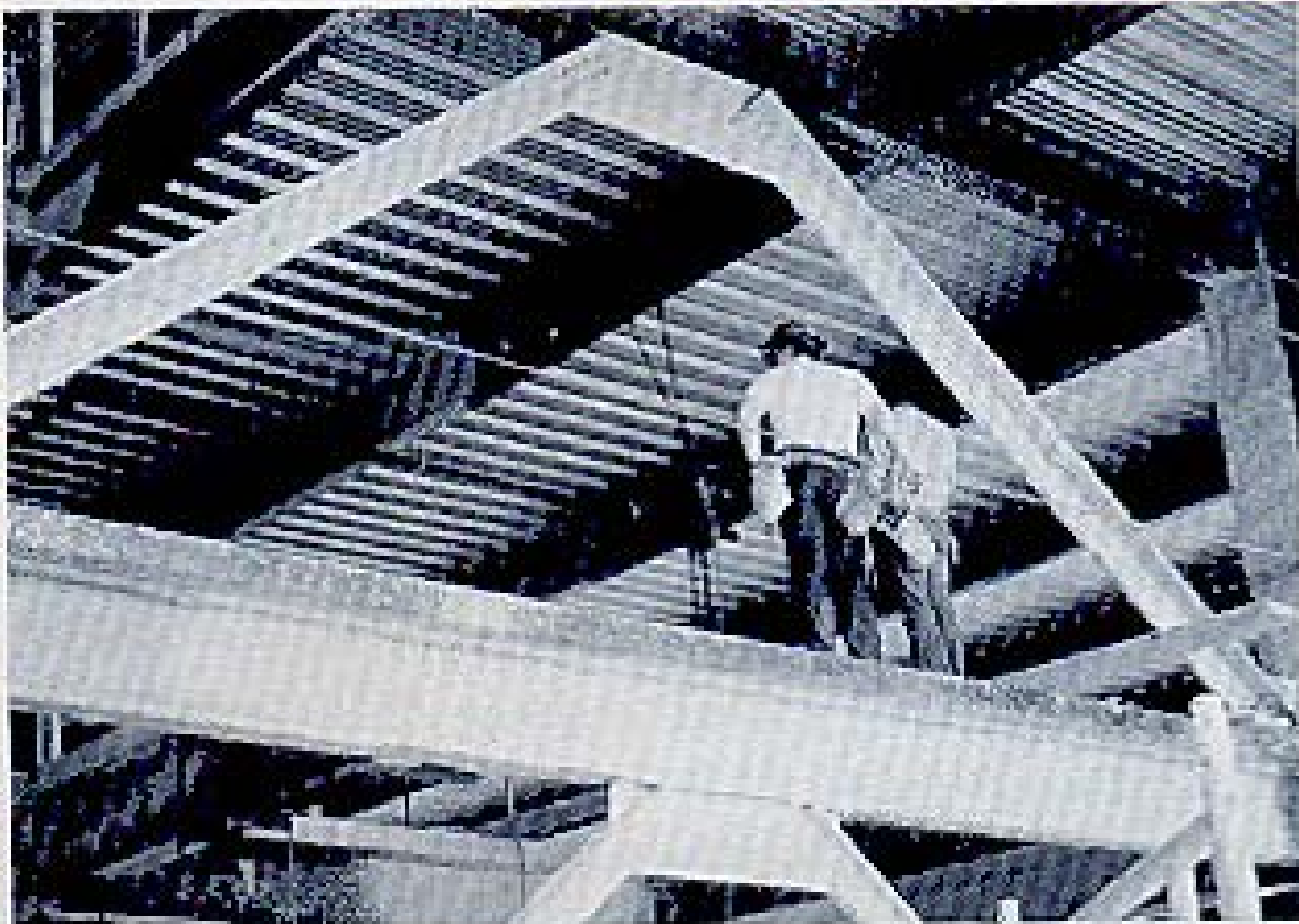
Figure 4.16 Inverted K bracing with double-angle connections.
