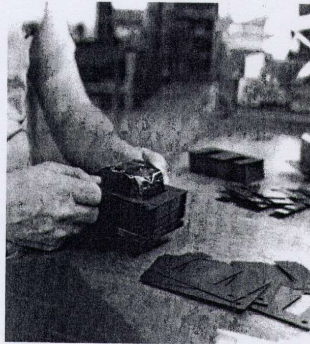
Figure 10.9b Stacking laminations inside a coil.
