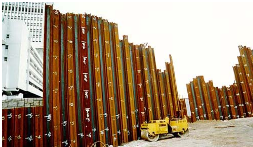
Sheet piles marked for driving
