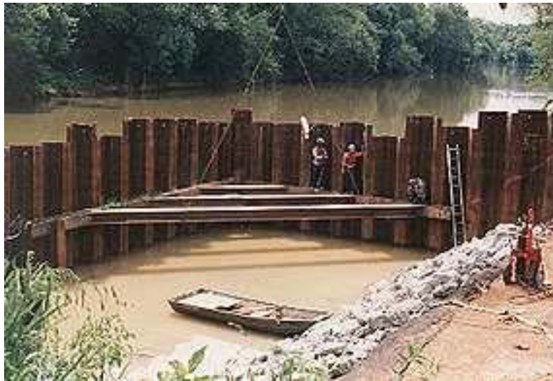
Sheet pile wall
