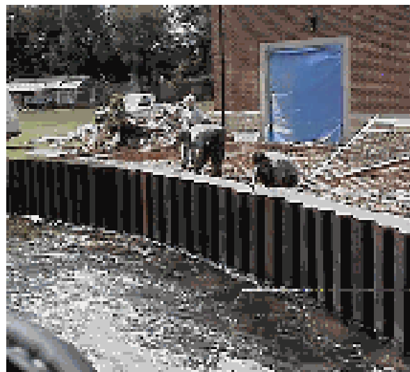
Sheet pile wall
