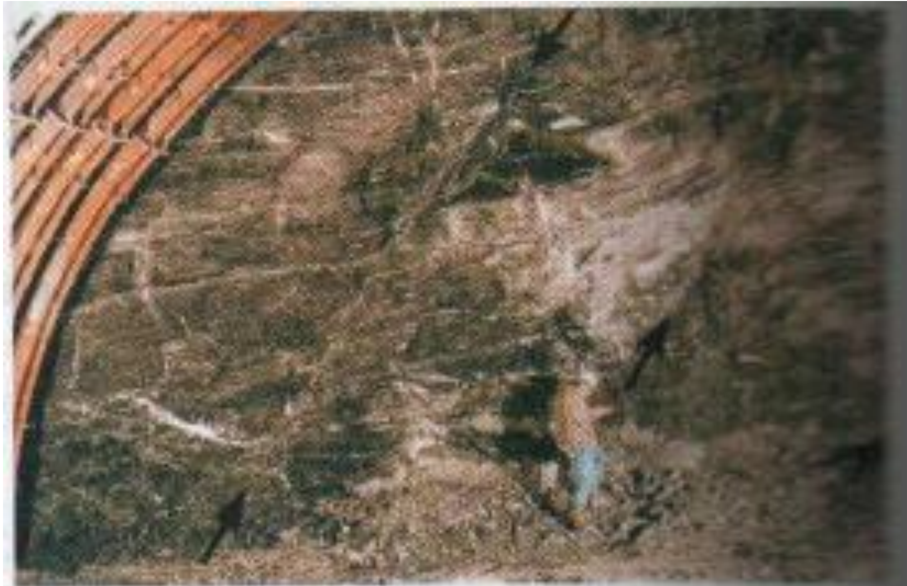
Figure 10.34 Faults intersecting the tunnel excavation face in RMR Class IV shales.
