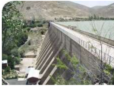
Fig 2: Ekbatan buttress dam (Iran)
