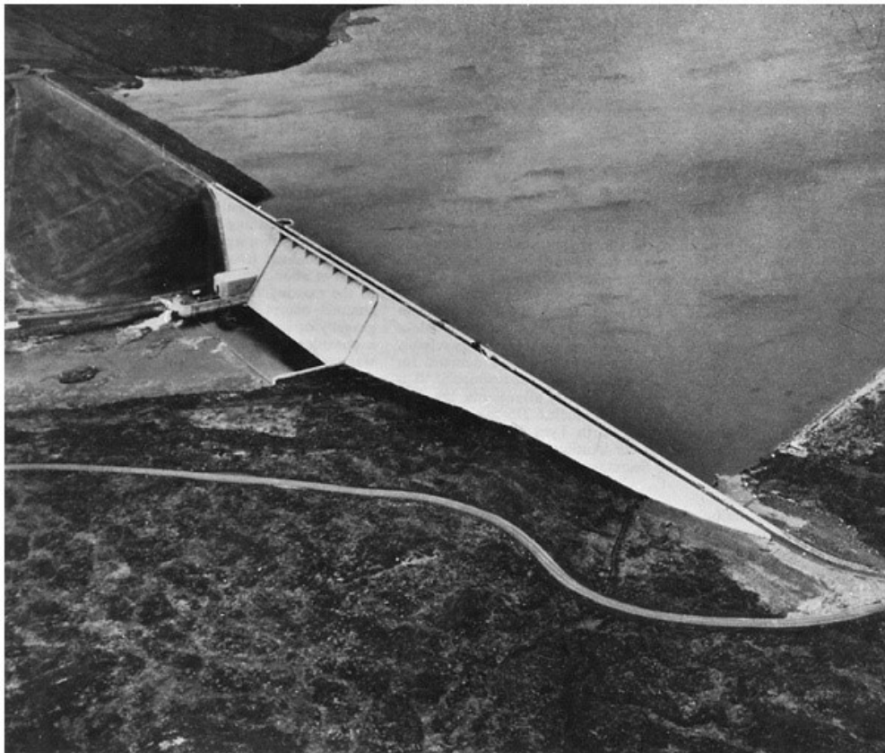
Fig 5: Cow Green Dam in Teesdale, northeast England, an example of a composite dam
