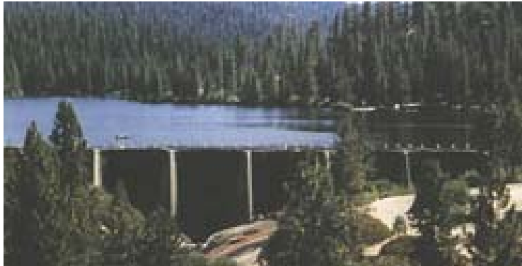
Hume Dam: Buttress dam
