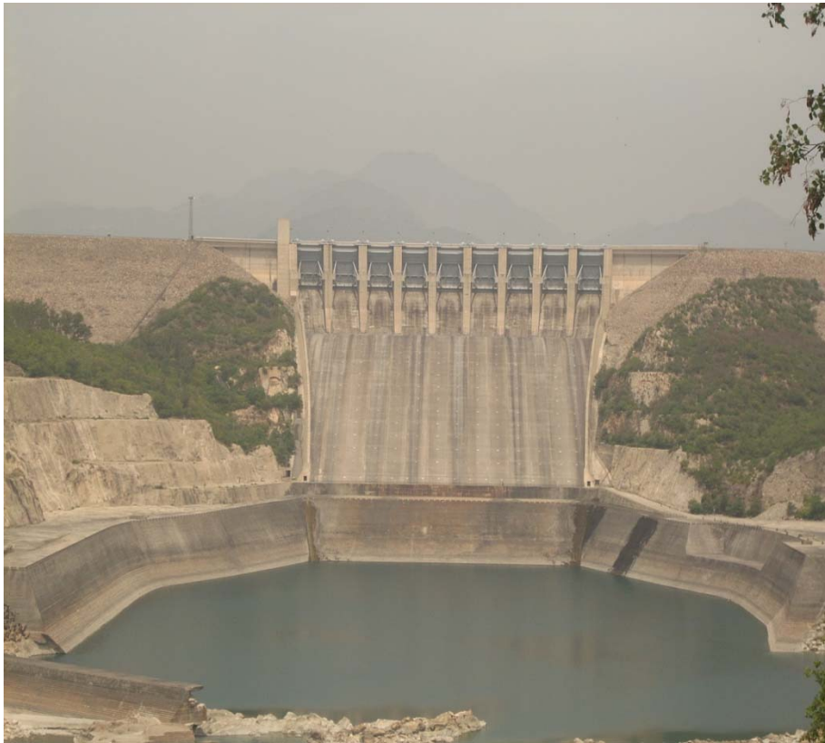
Auxiliary Spillway of Tarbela Dam
