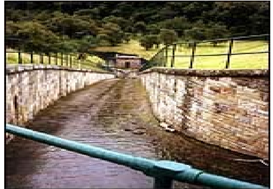
spillway chute from side channel to river
