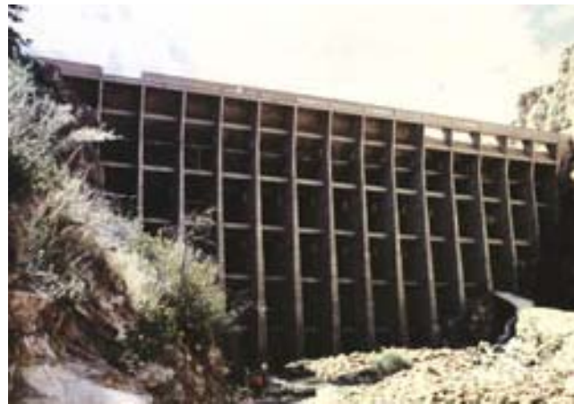
Le Prele Dam: Buttress dam
