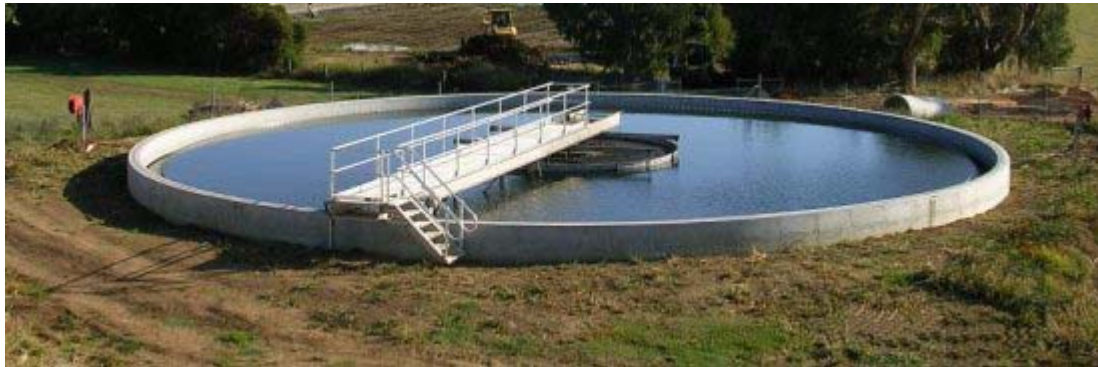
Figure 2-6: Primary settling tank
