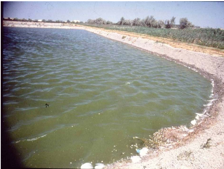
Figure 7. Embankment protection with stone rip-rap.
