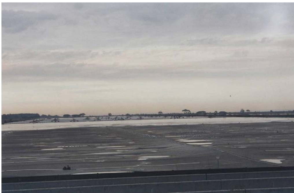
Figure 11. Covered anaerobic pond at the Western Treatment Plant in Melbourne, Australia.
