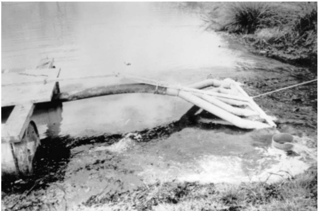
Figure 6.2 Pond desludging using a raft-mounted sludge pump. Detail: sludge suction head.
