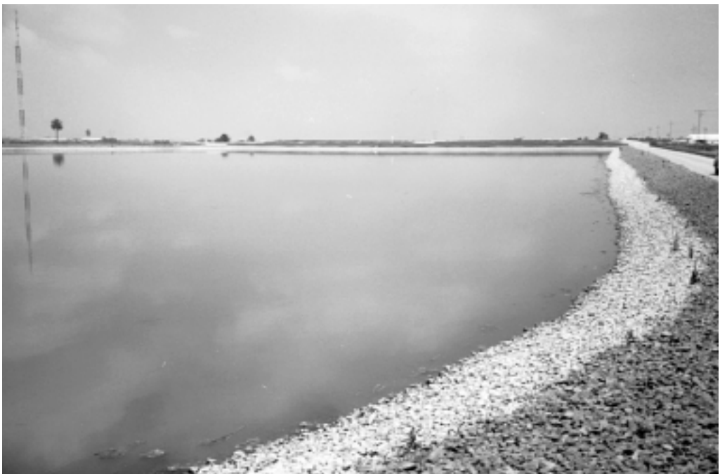
Figure 5.2 Embankment protection by stone rip-rap.
