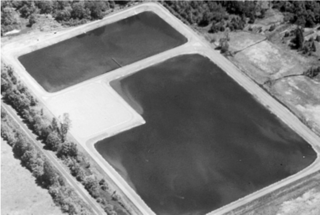
Figure 8.2 Rock filter installed in the corner of a pond at Veneta, Oregon, USA.
