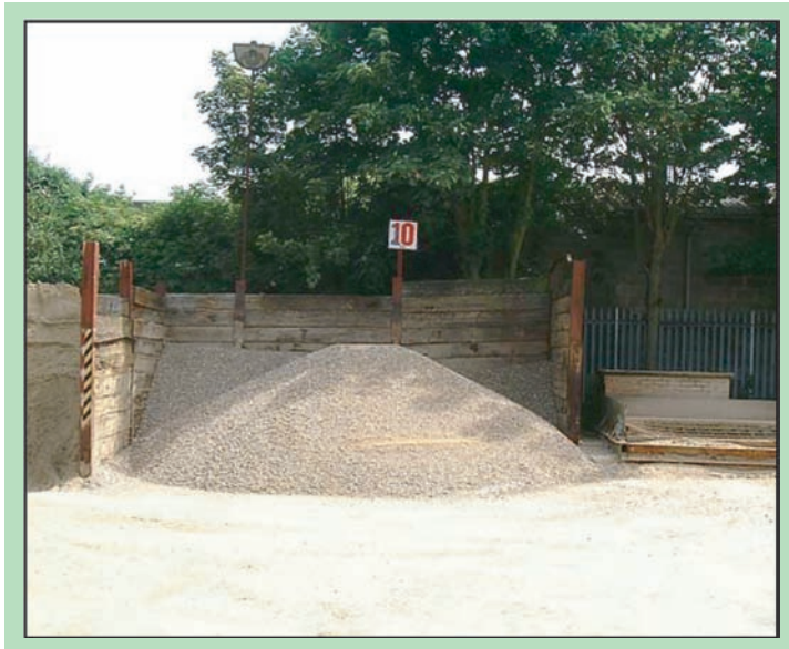
Figure 4.54 Coarse aggregate bin.
