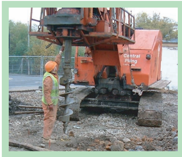
Figure 4.28 Crawling piling rig and auger.
