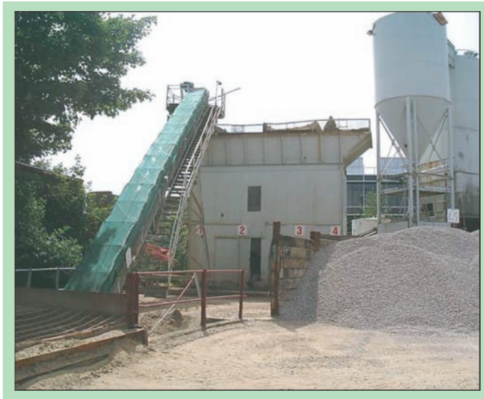
Figure 4.56 Conveyor and hopper heads.
