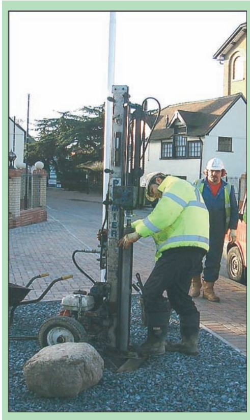
Figure 4.43 Drop hammer soil sampling.
