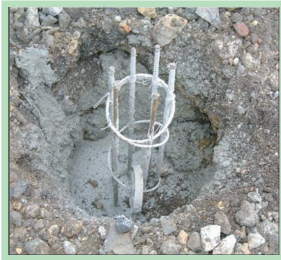
Figure 4.31 Pile cage ready to receive pile cap.
