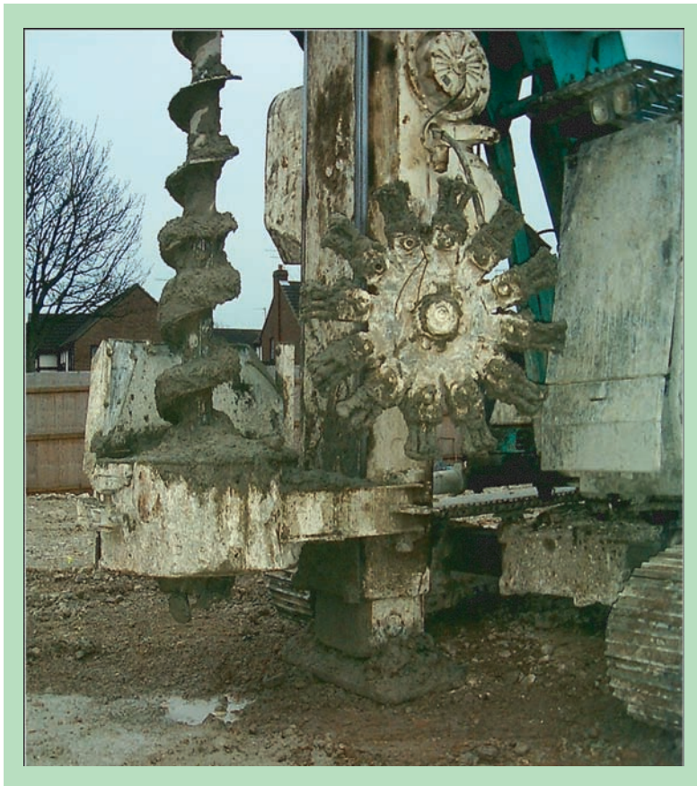
Figure 4.29 Piling auger and cleaning brush.
