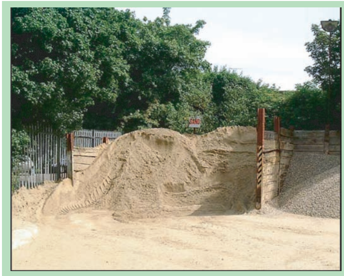
Figure 4.55 Fine aggregate bin.
