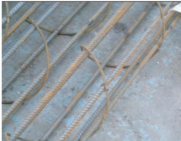
Figure 4.30 Pile cages.
