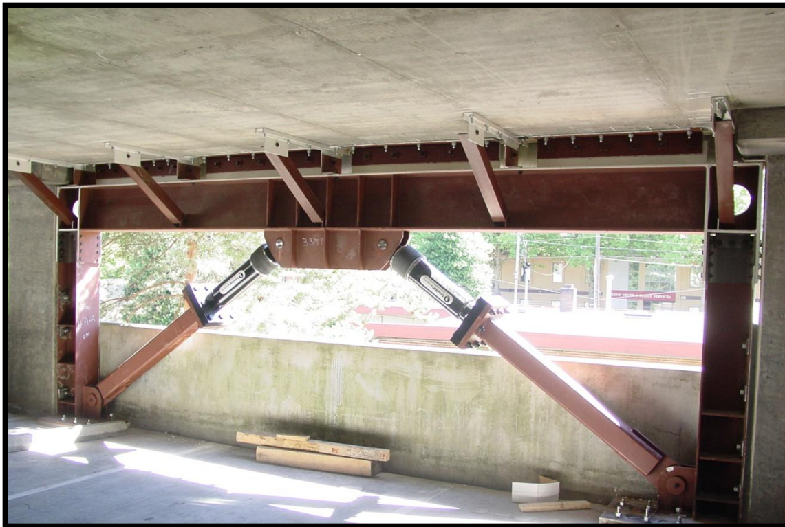
Viscous spring dampers
