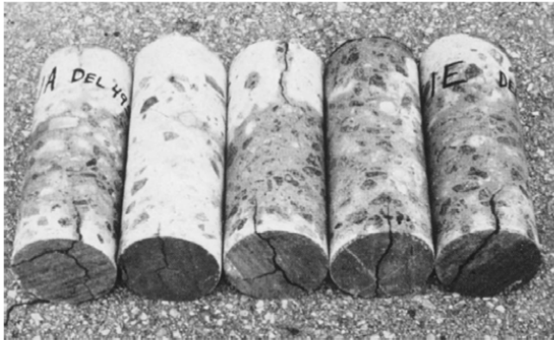
Pavement Cores Vertical Cracking
