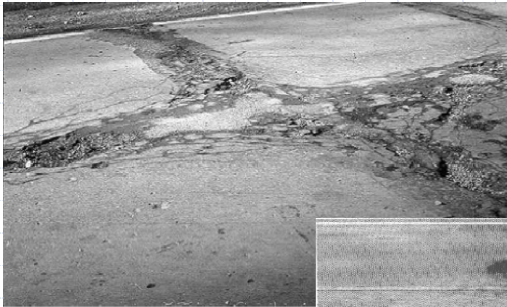
D-Cracking
