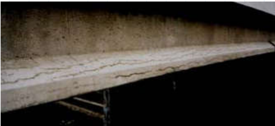
Map cracking in Wing Wall; surface discoloration around cracks
