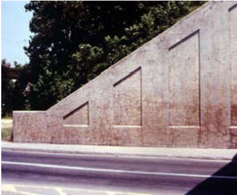
Map cracking in Wing Wall; surface discoloration around cracks
