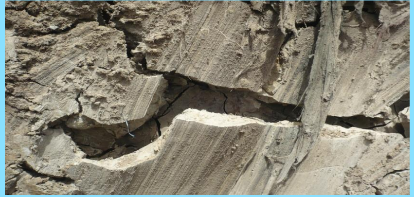
Shrinkage cracks at DG Khan Site
