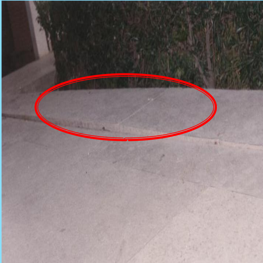
Lifting of floor slab due to Swelling of underneath soil
