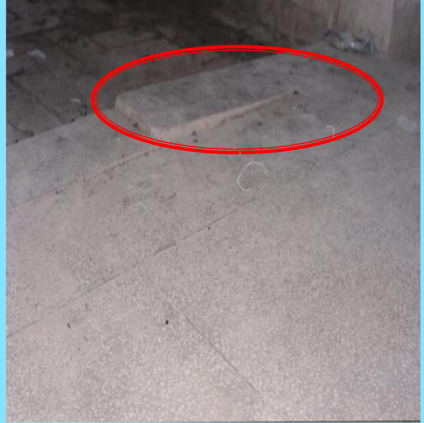
Lifting of floor slab due to Swelling of underneath soil
