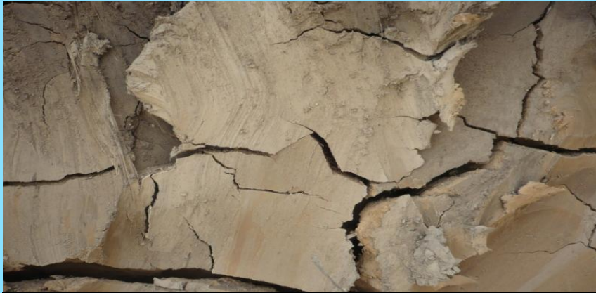
Shrinkage cracks at DG Khan Site
