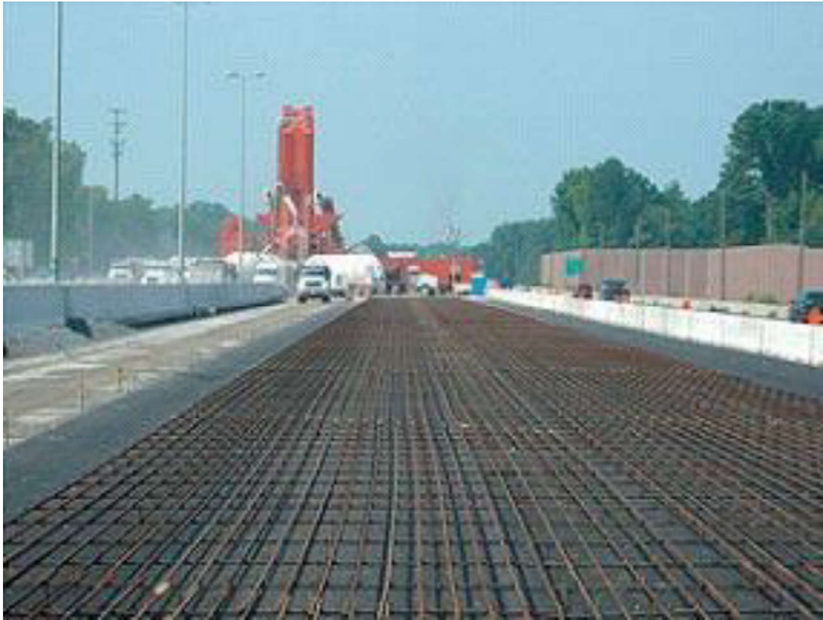
Continuously Reinforced Concrete Pavement (CRCP)
