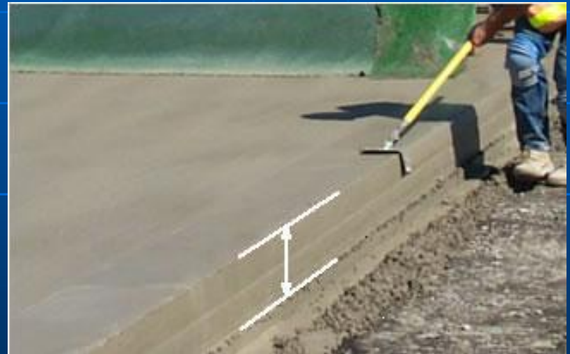
Rigid Pavement Slab (Surface Course) Thickness 36
